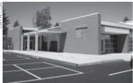
The new school addition relocated the administrative offices to a place where access can be better controlled.
