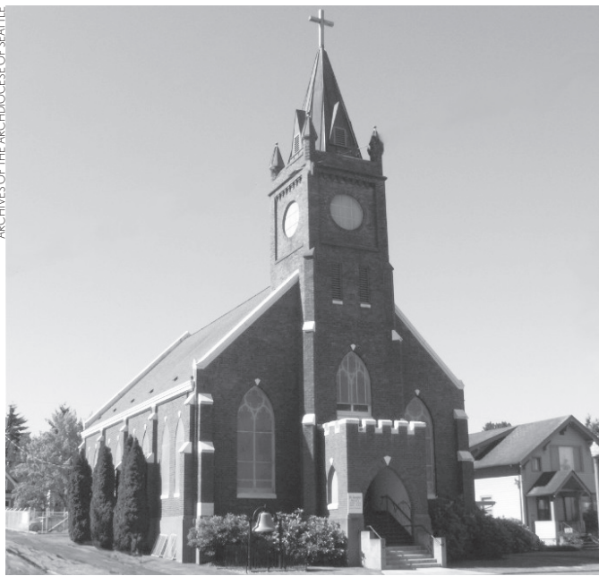
Except for the addition of a ramp and other minor changes, St. Joseph Church looks the same as it did 100 years ago. Its walls were made of "12-inch solid brick," longtime pastor Father Joseph Hayostek once boasted to the Tacoma News Tribune. Today the once all-Slavic parish welcomes all kinds of different nationalities, said Margaret Hofer, a member of the history committee.
